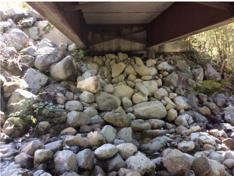
Left Bank Abutment when facing downstream
