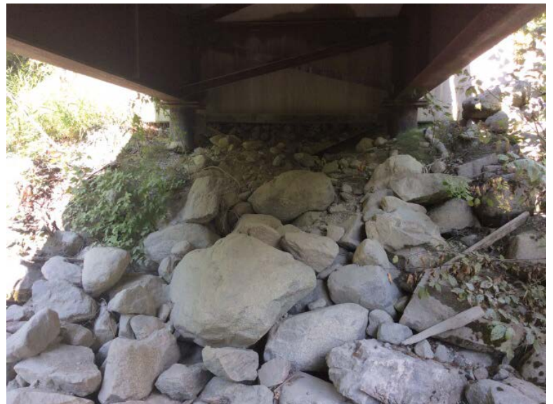
Right Bank Abutment when facing downstream
